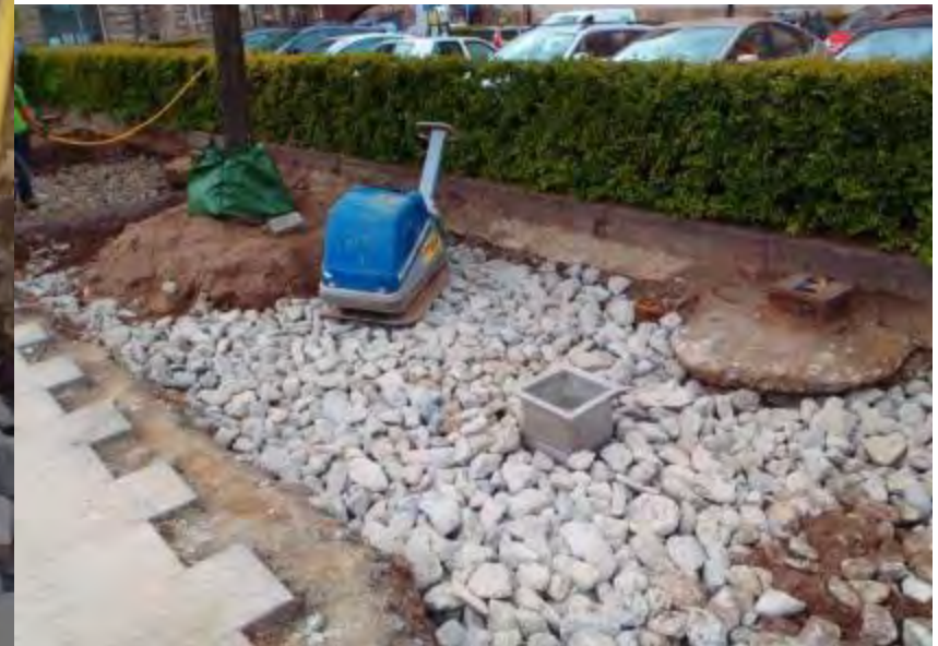
Recycled concrete used as a part of the structural soil instead of granite
