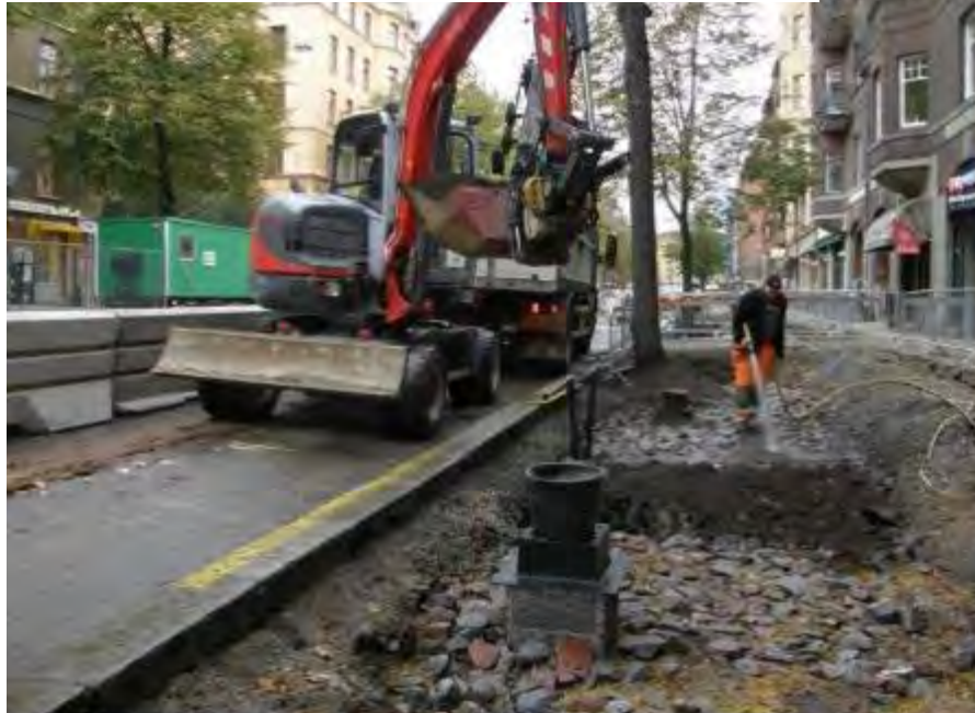
Flushing the soil into the structure
