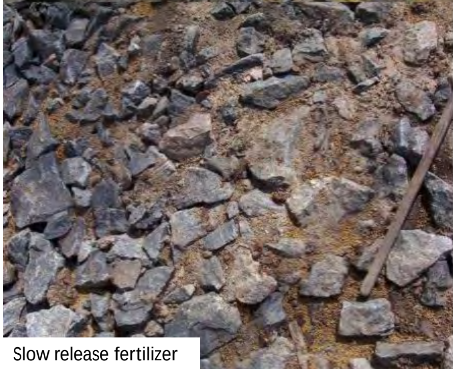
Layer for infiltration of rain water and aeration of the soil on top off the structural soil
