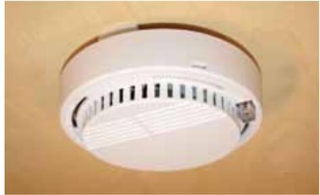
work must be installed in new housing units. The power supply of the device is ensured with a back up battery or accumulator.
