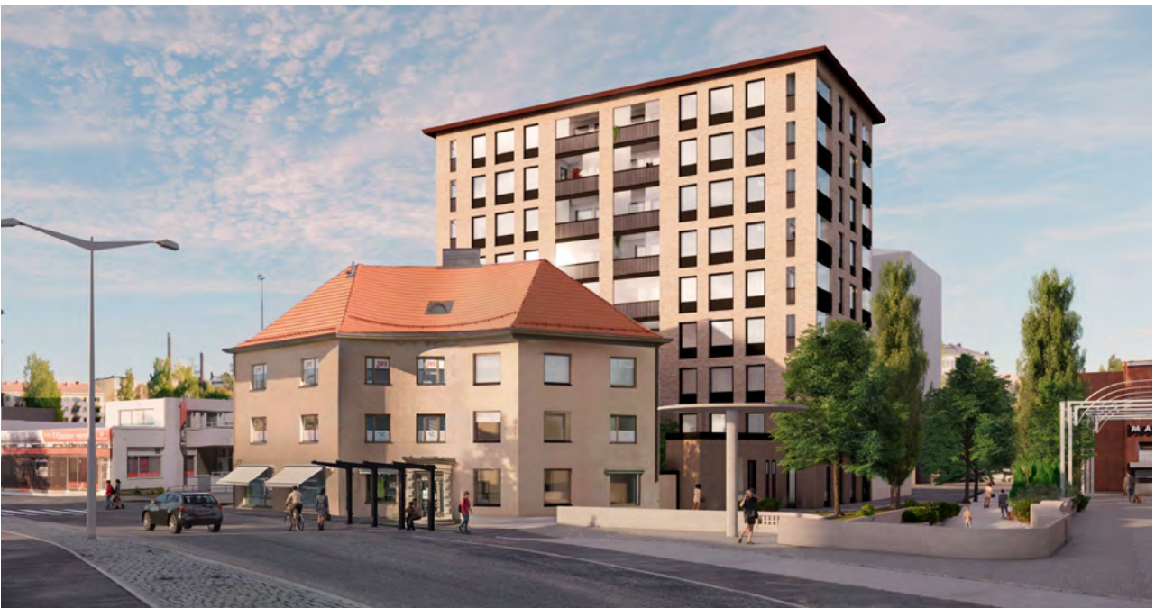
(106.) The building located along Kirkonkyläntie will be partially restored for residential use. A new residential building is being planned to replace the section that is to be demolished. © Arkkitehtipalvelu
