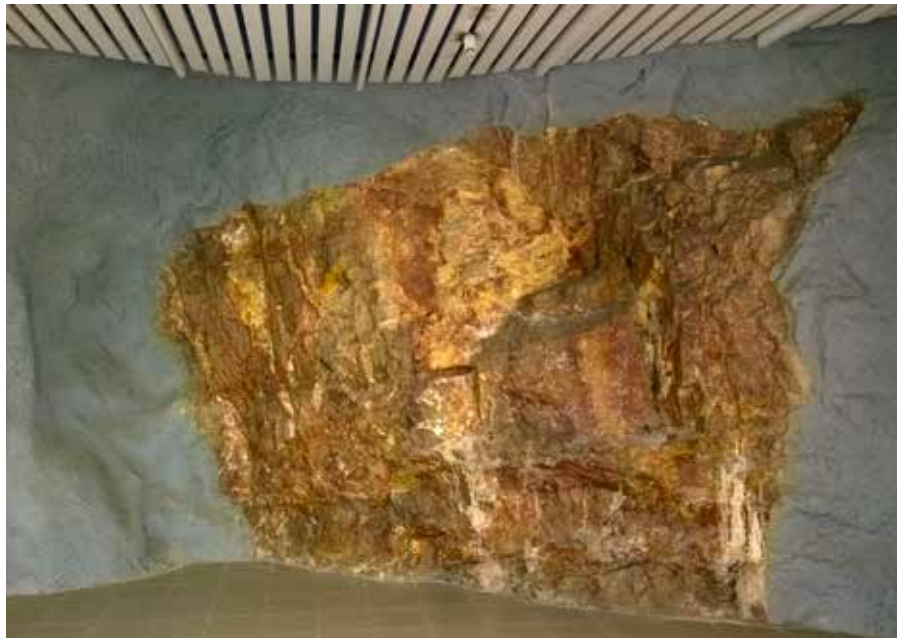
Fig. 2. A bare uncovered rock surface 'window' in the Kluuvi underground parking hall in Helsinki. (Photo: Ilkka Vähäaho)
