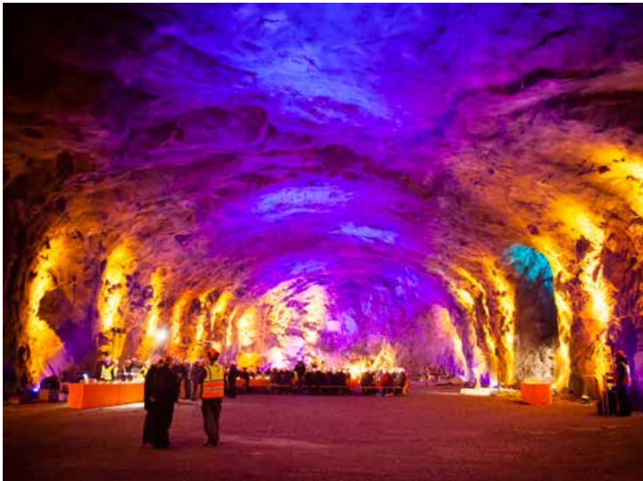
Fig. 24. The cold water reservoir for district cooling in Helsinki's city centre was built between 50–90 metres from ground level because of the lack of free underground space. (Photo: Helen Oy)
