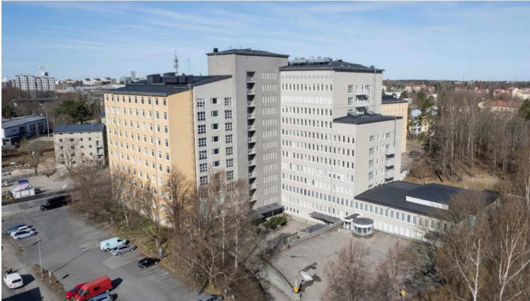
Photo 5 The maintenance yard is at an elevation of about 8.8 m
