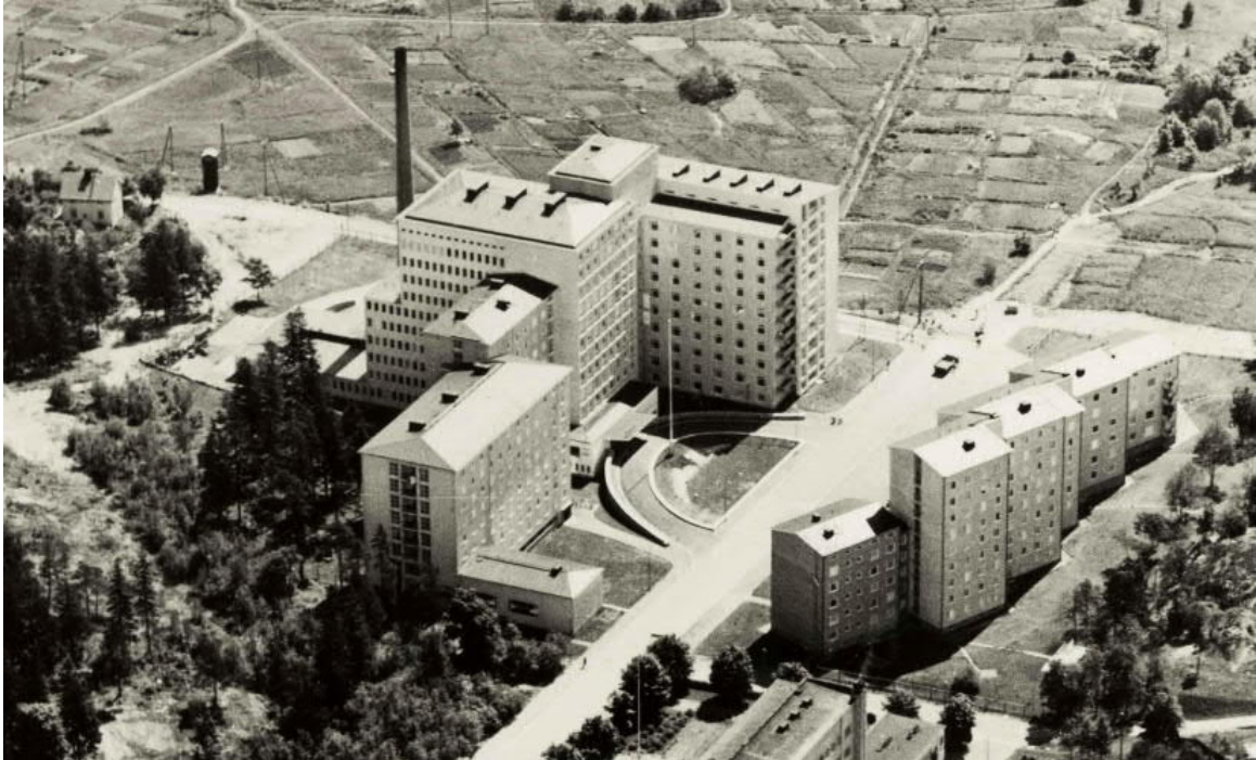
Photo 3 The architectural history of Kättilöopisto Maternity Hospital is appended to the competition programme
