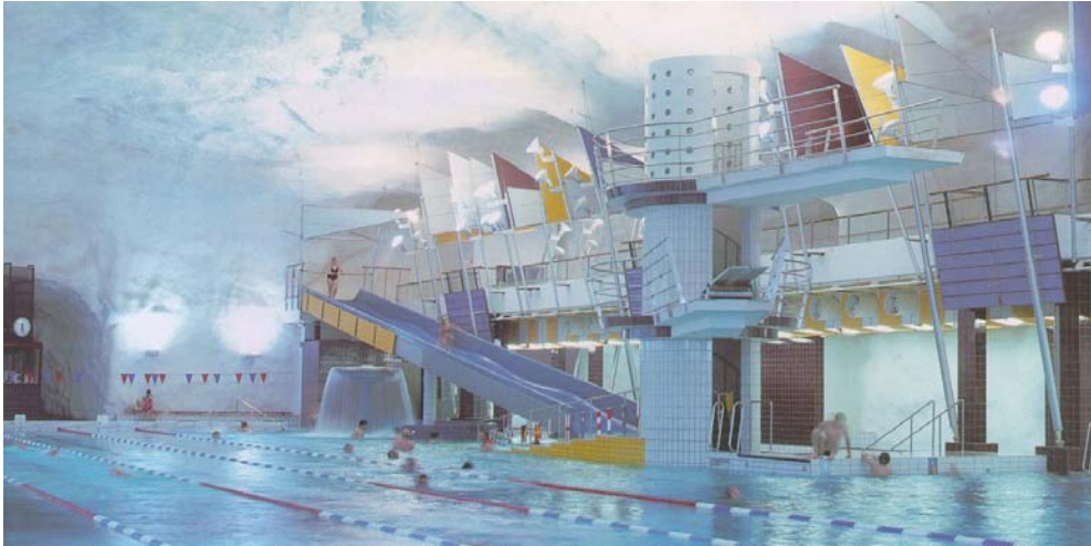
Fig.2. Underground Swimming Pool in Itäkeskus which can accommodate 1,000 visitors at a time and can be converted into an emergency shelter for 3,800 people if necessary. (Photo: Erkki Makkonen).
