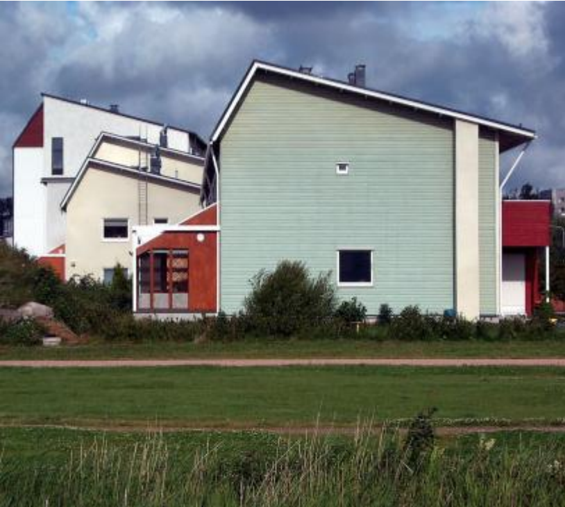
The roof forms contribute to the 'eco-architecture' image in Eco-Viikki.
