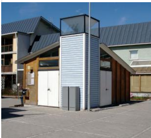
The refuse bin store at Versokuja 4 helps to demarcate the street line.
