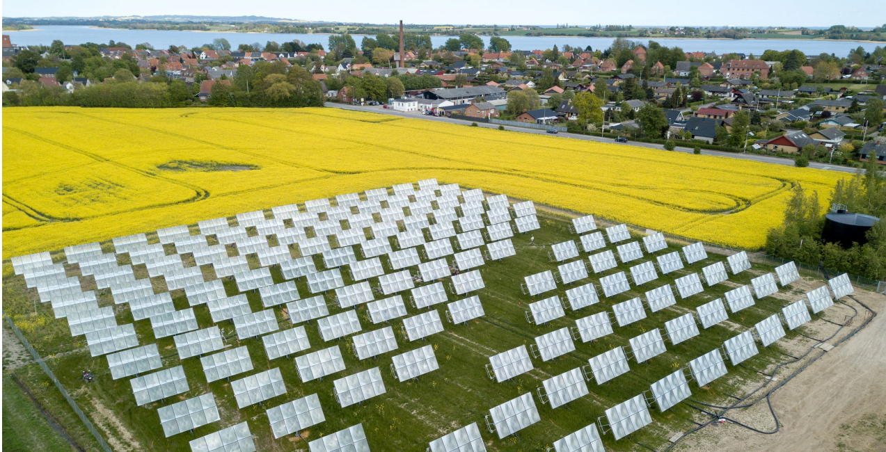
Figure 3- Large scale concentrating collector field as part of a district heating network.
