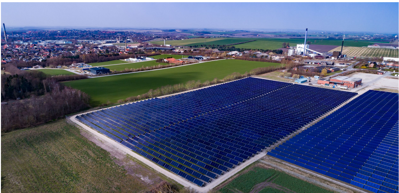
Figure 2- Large scale flat plate collector field as part of a district heating network
