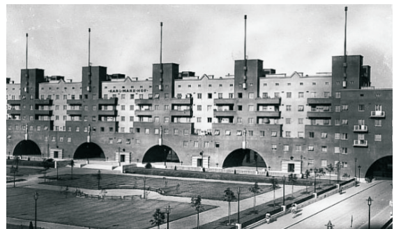
One of the most prominent examples of Red Vienna’s “Kommunaler Wohnbau” (Communal Housing): the “Karl-Marx-Hof” (19th district of Vienna).
