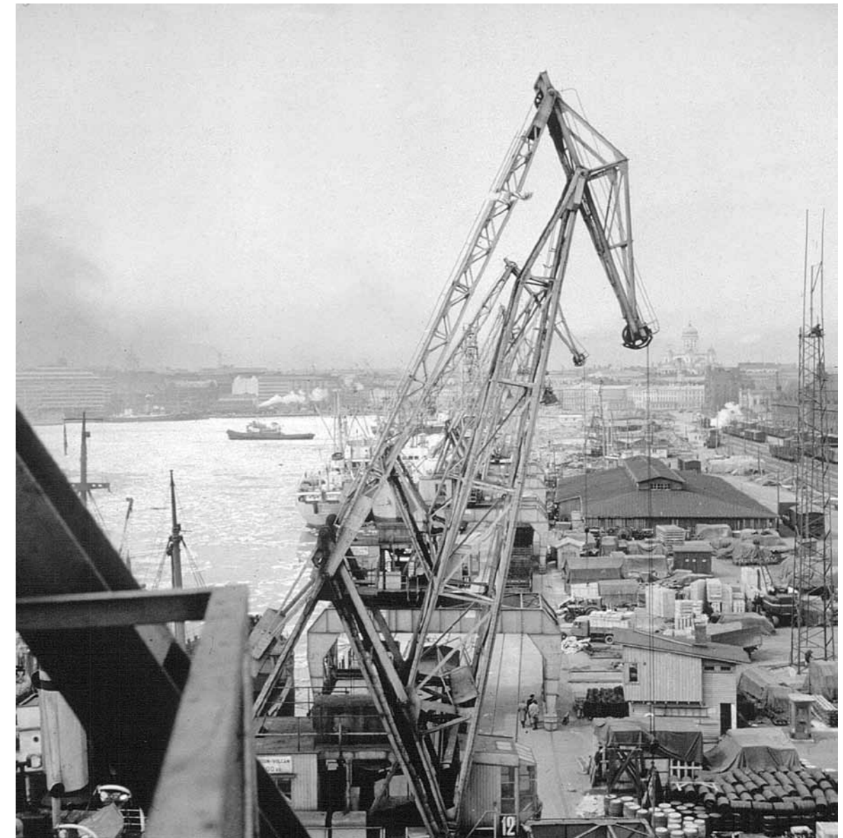
FIGURE 2. Cranes, goods and trains at the Katajanokka pier in Helsinki South Harbor in 1957, with the iconic neoclassical facade of the city to the sea in the background. Photo: K. Laitila, Helsinki City Museum.
