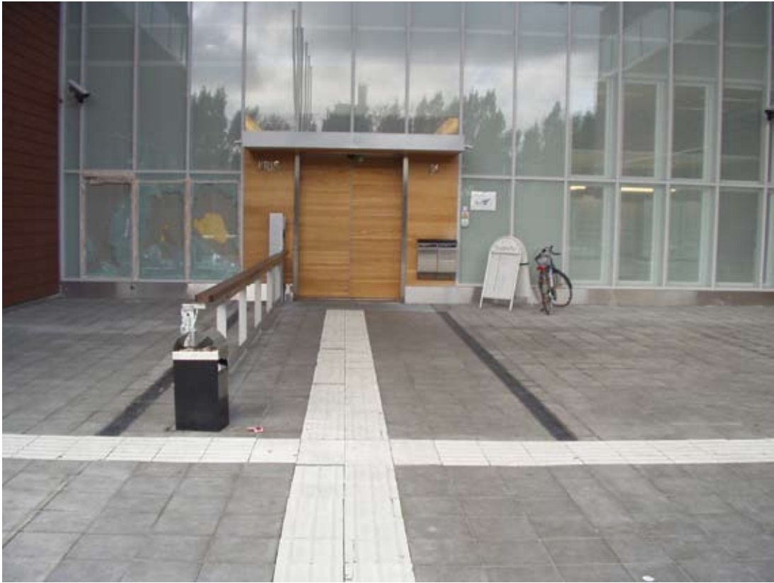
Figure 5: The environs of Iiris, the office of the Finnish Federation of the Visually Impaired, are at the demanding level of special accessibility, with particular attention paid to mobility guidance for people with visual impairment.
