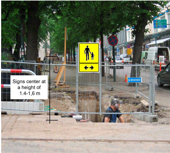
Figure 3. Worksite signs or their mounting posts/bases must not cause a risk of collision, falling or tripping.
