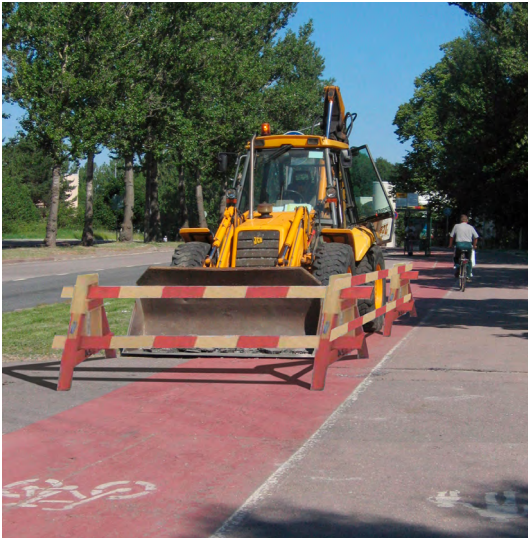
Figure 2. Protection of worksite machinery must not force pedestrians to use the carriageway.
