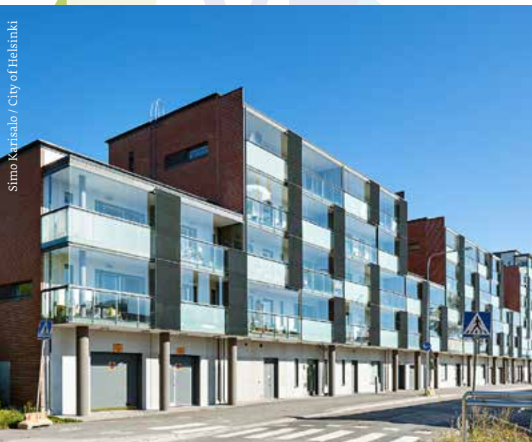
Hernepellontie 26 low-energy apartments
