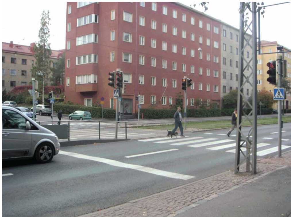
Figure 37: A recessed stop line at a signalised zebra crossing in Helsinki.
