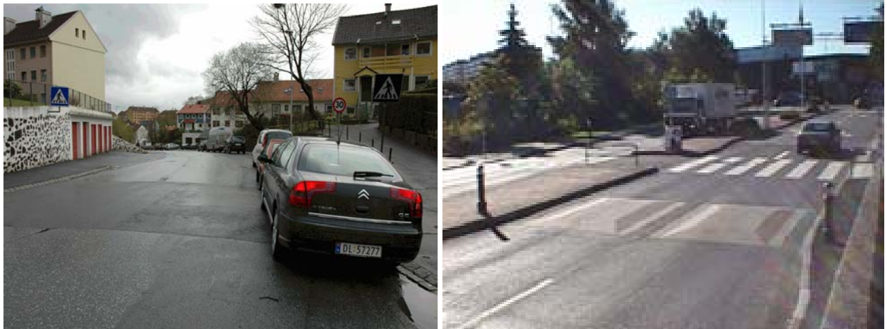
Figure 32: A hump of asphalt in Bergen and the Swedish concrete element (Måsen).
