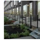
Pacific Cannery Lofts Oakland, CA David Baker and Partners https://www.tippingstructural.com/projects/project_details/31#
