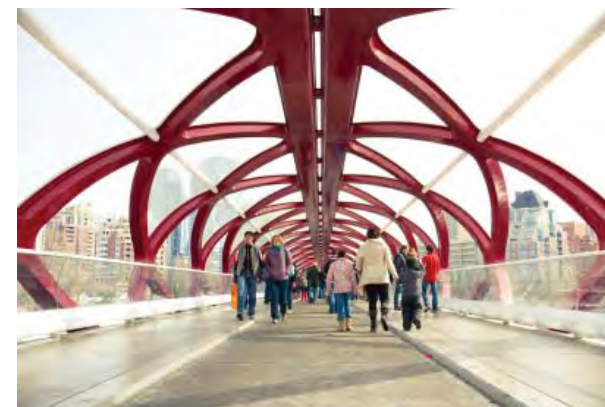
Calgary pedestrian bridge
