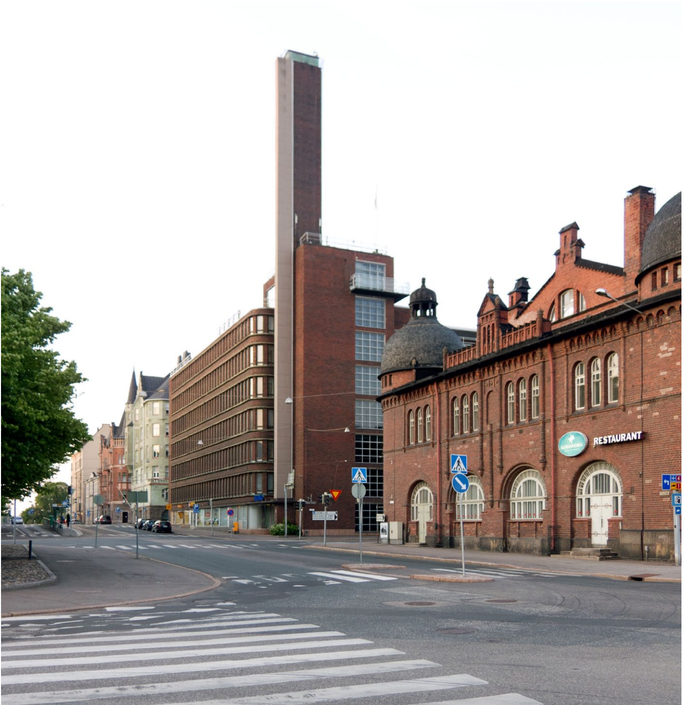
View from the north-east corner of the site at the intersection of Katajanokanlaituri and Satamakatu looking north toward the custom & warehouse building and the Kesko headquarters beyond.
