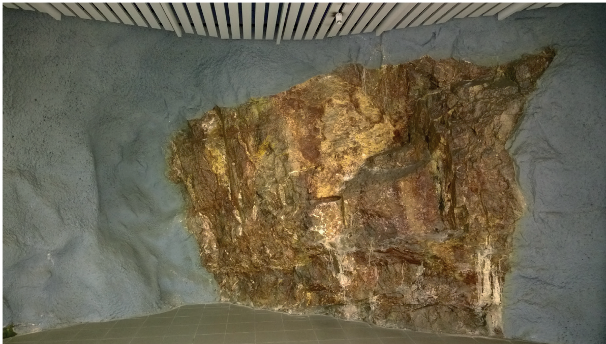
▲ Fig. 2. A bare uncovered rock surface 'window' in the Kluuvi underground parking hall in Helsinki (Photo: Ilkka Vähäaho).
