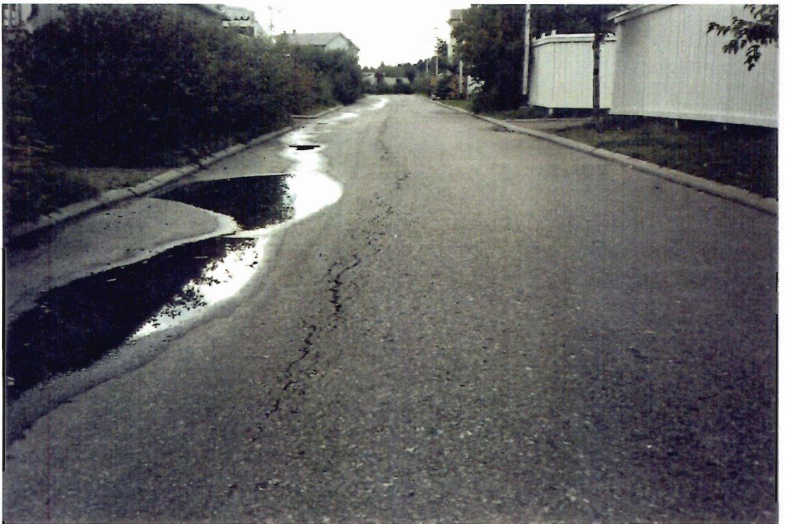
Figure 15. Thaw Settlements observed in Torpparinmäki area of Helsinki in summer 1987.
