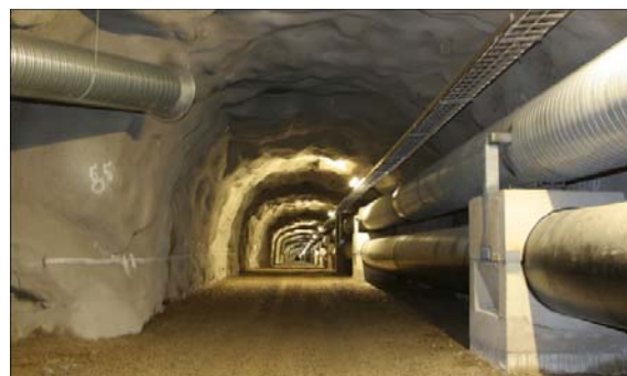
Fig. 9 Typical Utility Tunnel (Photo: Jorma Vilkmán)
