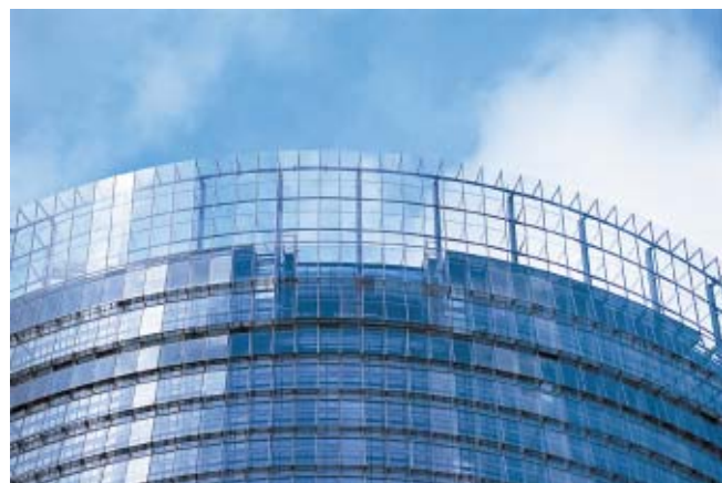
Fig 6 High terrace and wintergarden
