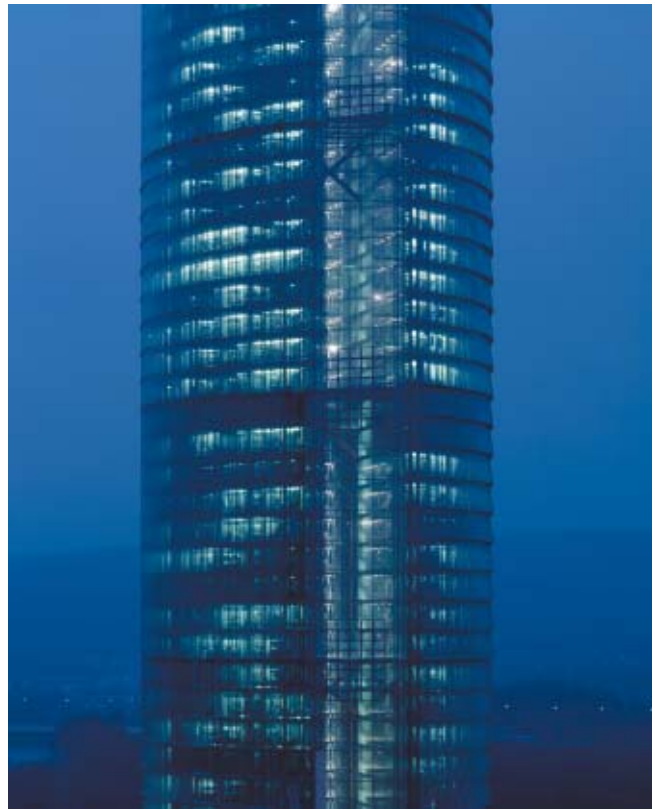
Fig 11 View of the Post-Tower at night
